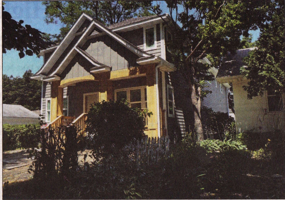
With the proposed new limits on height and lot coverage and requirements for architectural details on sidewalls, this new home under construction in the 1600 block of James Avenue may have needed variances.
